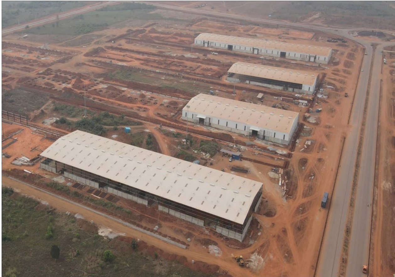
Warehouses under construction - GDIZ
